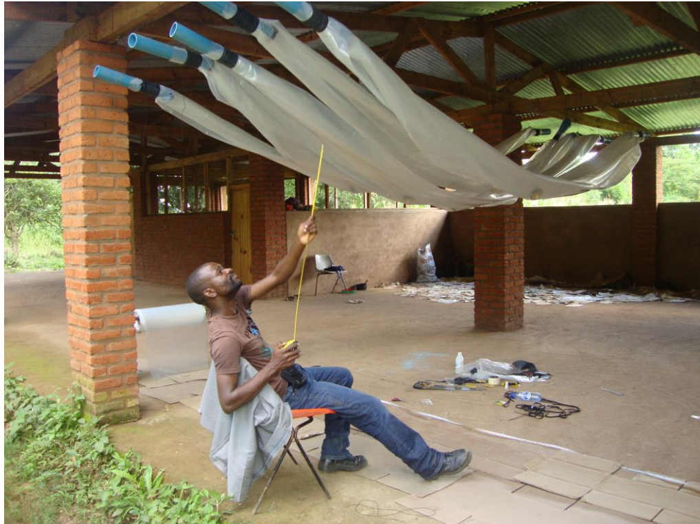
Figure 5: Assembled polyethylene tubes hanged to the roof for safe keeping before installation
