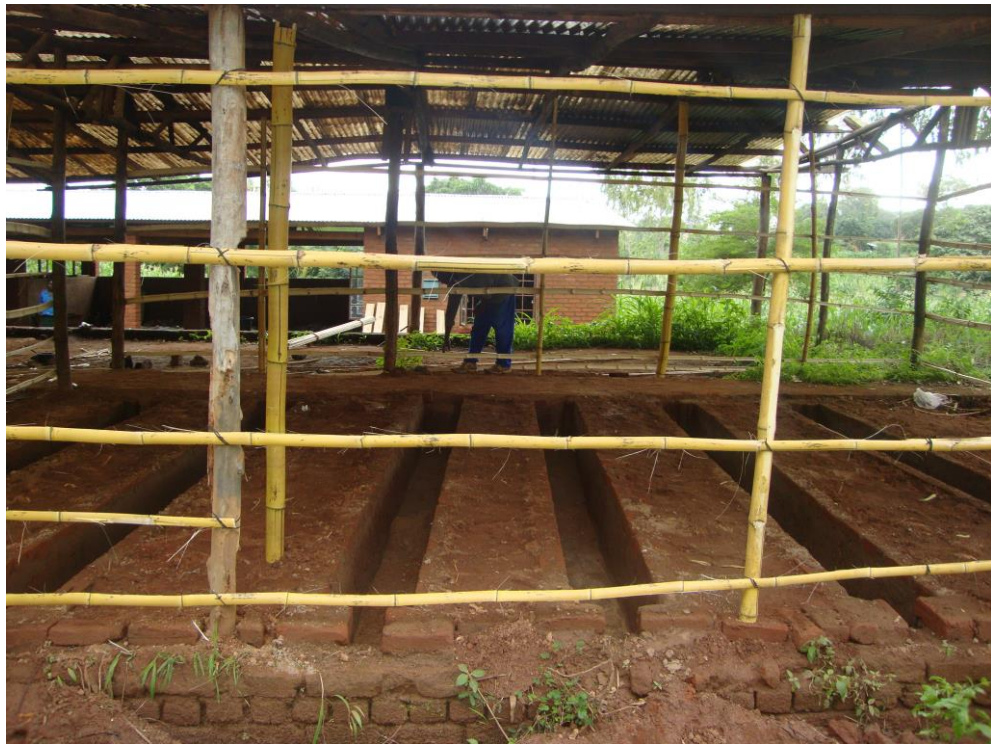
Figure 4: Completed trenches inside a bamboo enclosure at the project site
